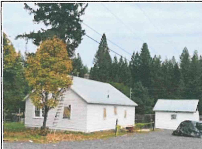
NRC House #3 is now protected with a fresh coat of primer/sealer. It awaits interior renovations to make it usable for partnership programs with SOU and other extended learning programs.
