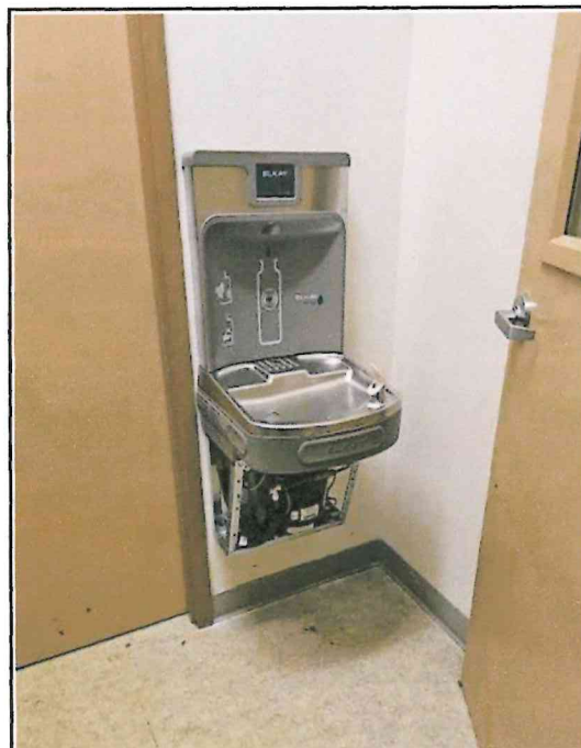
Thank you to Mr. Childers for installing our new drinking fountain/bottle filler by the entrance to the gym concession stand! This drinking fountain delivers fresh water from our local Ginger Springs. 12/26/23
