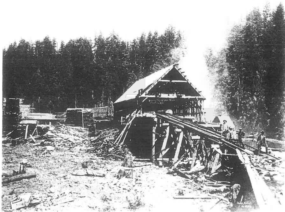
Figure F : The Sawmill Seen from the Southwest (ca. 1904)
