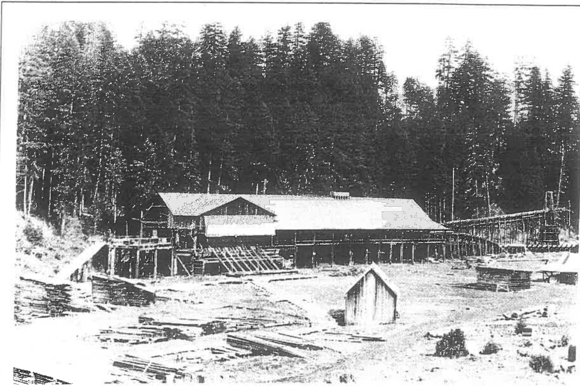
Figure I: Overview of Sawmill, Seen from the Northwest
